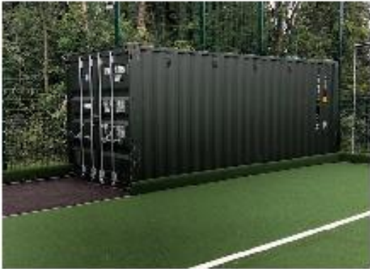
Maintenance equipment store
