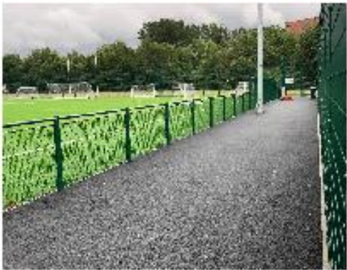
Porous macadam hardstanding to side of pitch
